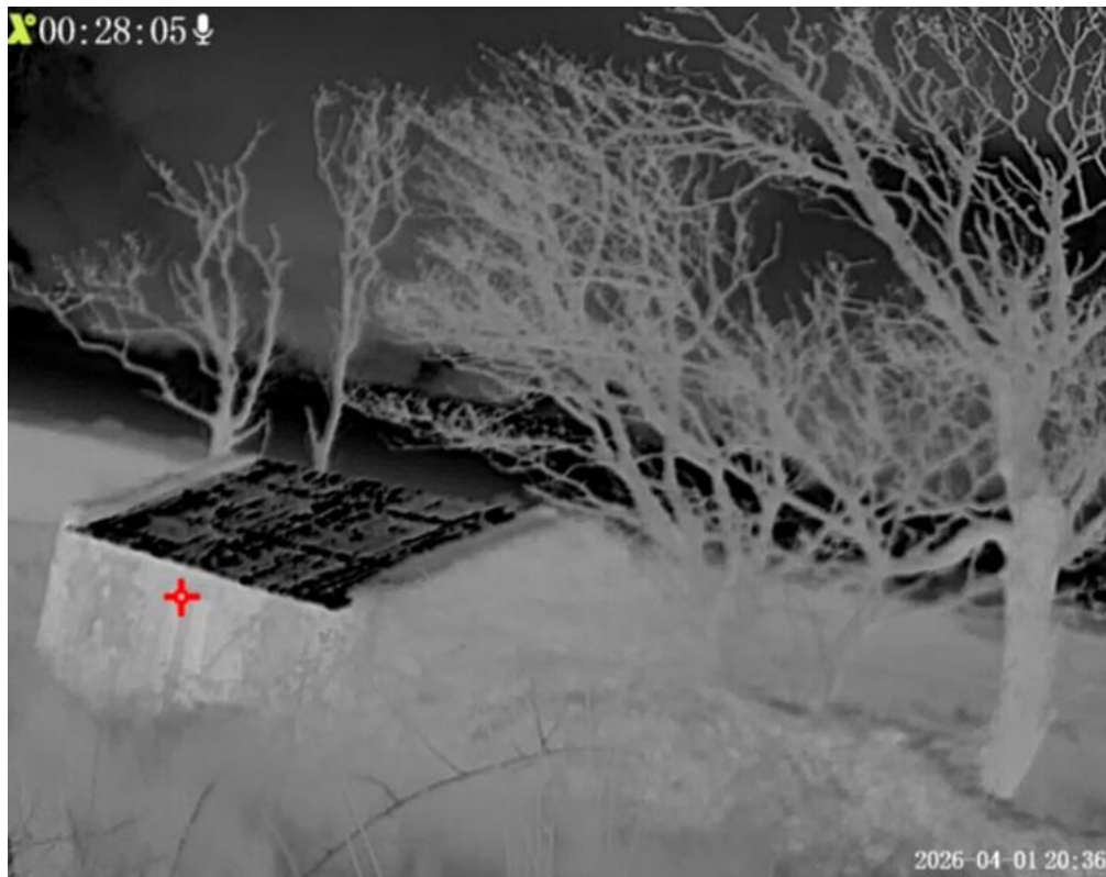
Plate 1: Building 59, trees no 28, 30 & 32
